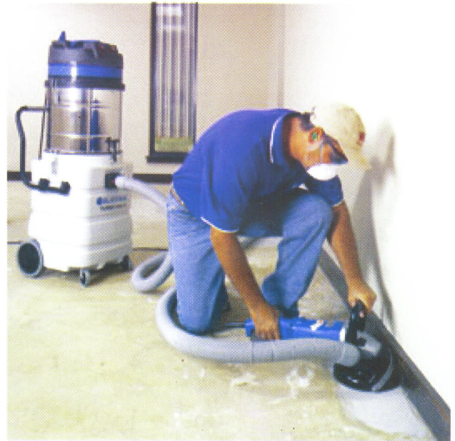
7" Grinder Assembly with Convertible Shroud Up
